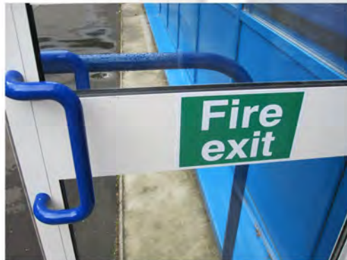
Colour contrasting doors, frame and handles for DDA purpose
