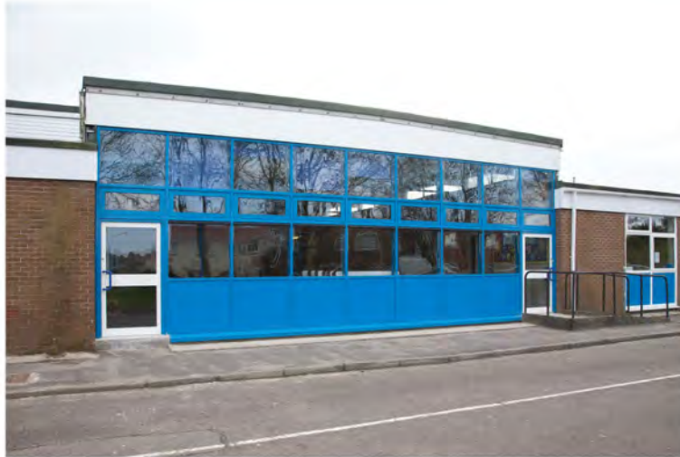
The new curtain wall
