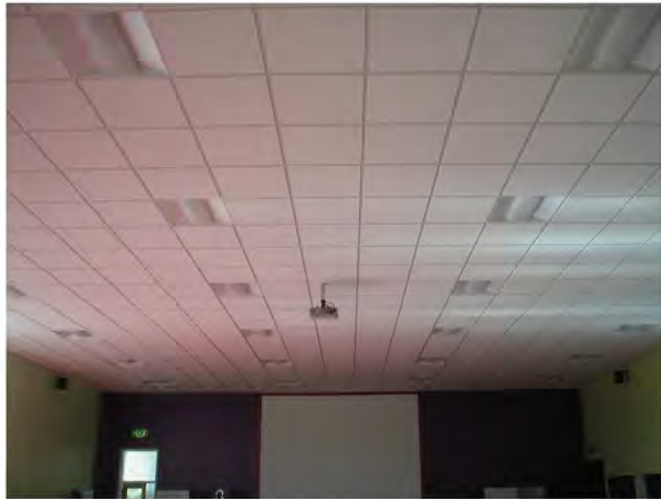
Photo showing the new ceiling
