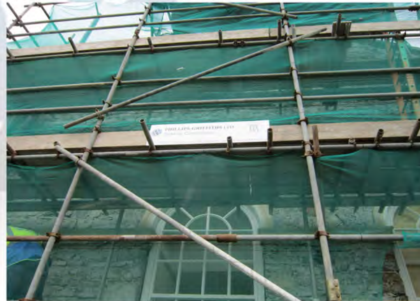
Scaffolding up and render removed
