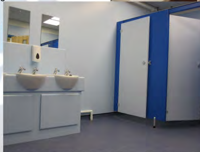
The completed toilets with a clean fresh look
